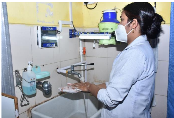
Facility staff observing all recommended steps of handwashing with the help of Datakalp SafeHands AI machine, at District Hospital, Mahasamund
