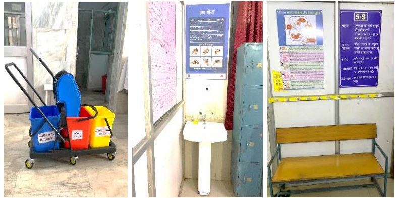
WASH infrastructure at the facility (L-R): 3-bucket mopping trolley and WASH information, education, and communication posters placed strategically around the facility.
